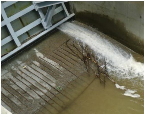
**b. Damage to sediment sluice, requiring periodic repair of steel gate seat and replacement of granite blocks**
